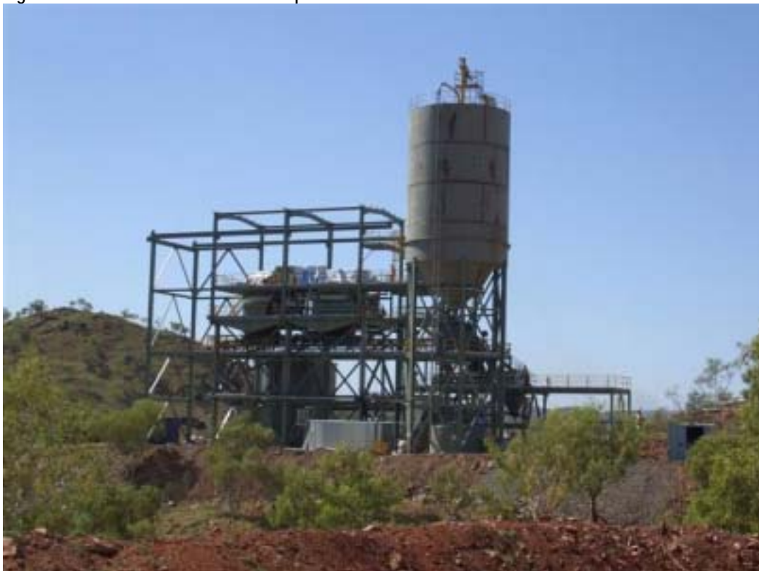
Figure 1: Paste Plant construction at September 2007
