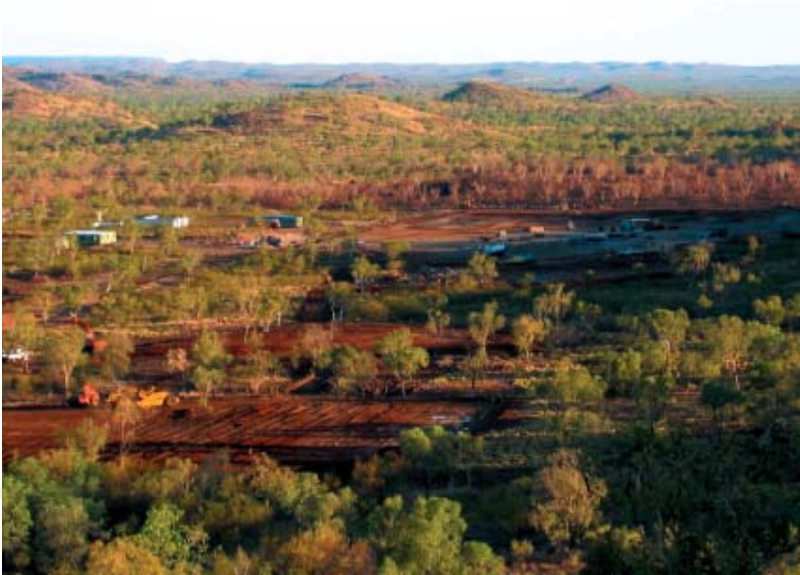
Figure 1 - Sally Malay Plant site earthworks, September 2003
